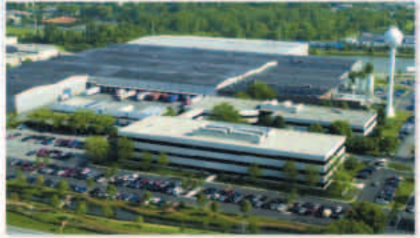
Medline corporate headquarters and manufacturing facility in Mundelein, IL.
